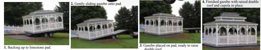
1. Backing up to limestone pad.
